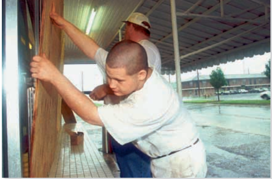
Figure 17 The people in this picture are preparing for a hurricane. The wooden boards help protect their windows from the high winds of a hurricane.
